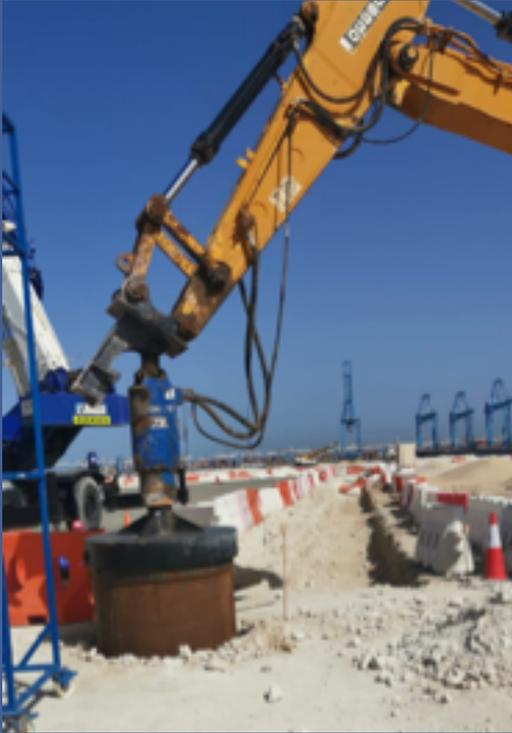
The 1200mm casing with auger was positioned at the drill point and was driven into the ground. Once set in the ground, the casing top adaptor plate was unlocked, and the auger was inserted in and the isolated soil inside the hole was drilled out.
